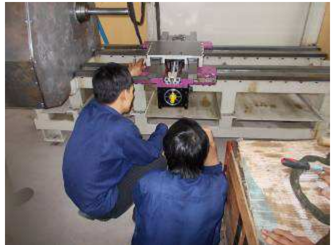
Photo 15: The X engine fitted done.
