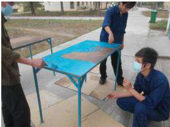
Photo 7: Diligently painted. As the plates were partially somewhat oily already, since they had been in use for 2 years, the project was not as easy.
