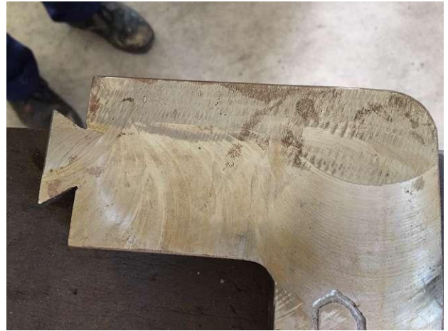
These traces of too rapid feed will not go away by galvanizing. That must be welded or discard the clamp.
