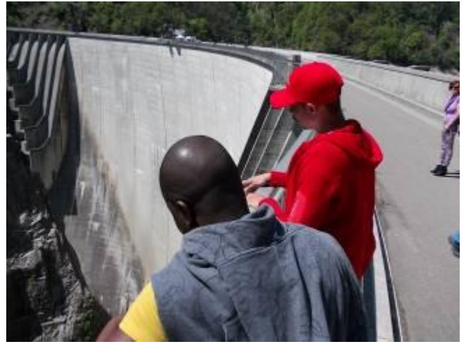
P36 Very high wall, the dam Versasca.
